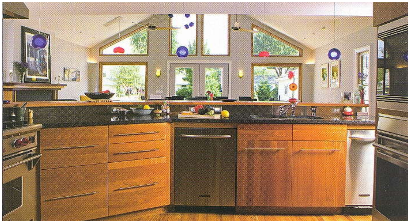
Above: On the kitchen side of the bar, Wayda's "appliance envy" was soothed with the French-top Wolf Range, wall microwave and convection oven, dishwasher and trash compactor and, not visible, a large refrigerator/freezer. Their old kitchen had a small, underpowered gas stove and no dishwasher. Opposite: Exotic purpleheart wood, which Wayda says is "a weed tree" in South and Central America, was incorporated in the floor of the dining area.
