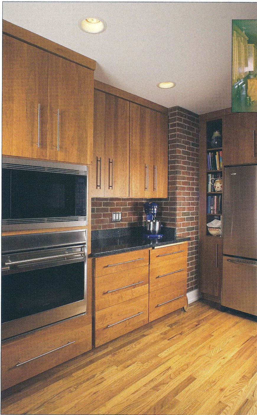
Thin brick was applied like tile to the kitchen walls, and oak flooring was installed to match the rest of the house. Davis uses the baking counter at center to make pies.
